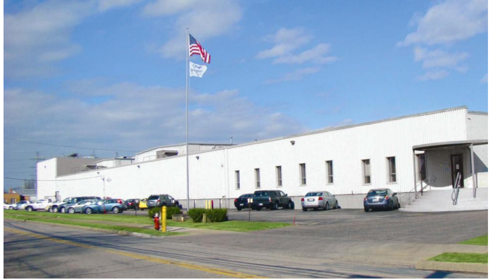
Figure 2: Image of AG Cleveland Facility
