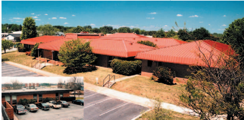
Butler non-residential metal roofs are known for their longevity, durability and aesthetics, making them the high-quality option for many re-roofing projects, such as this one at the Anderson Mental Health Center in Anderson, S.C.
